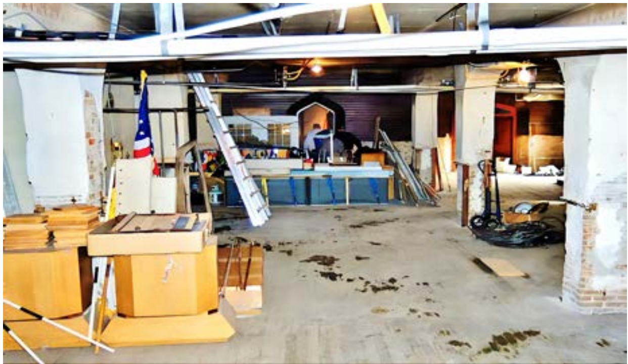
Basement prior to renovation, Saint Joseph Church, Marysville, January 22, 2007
