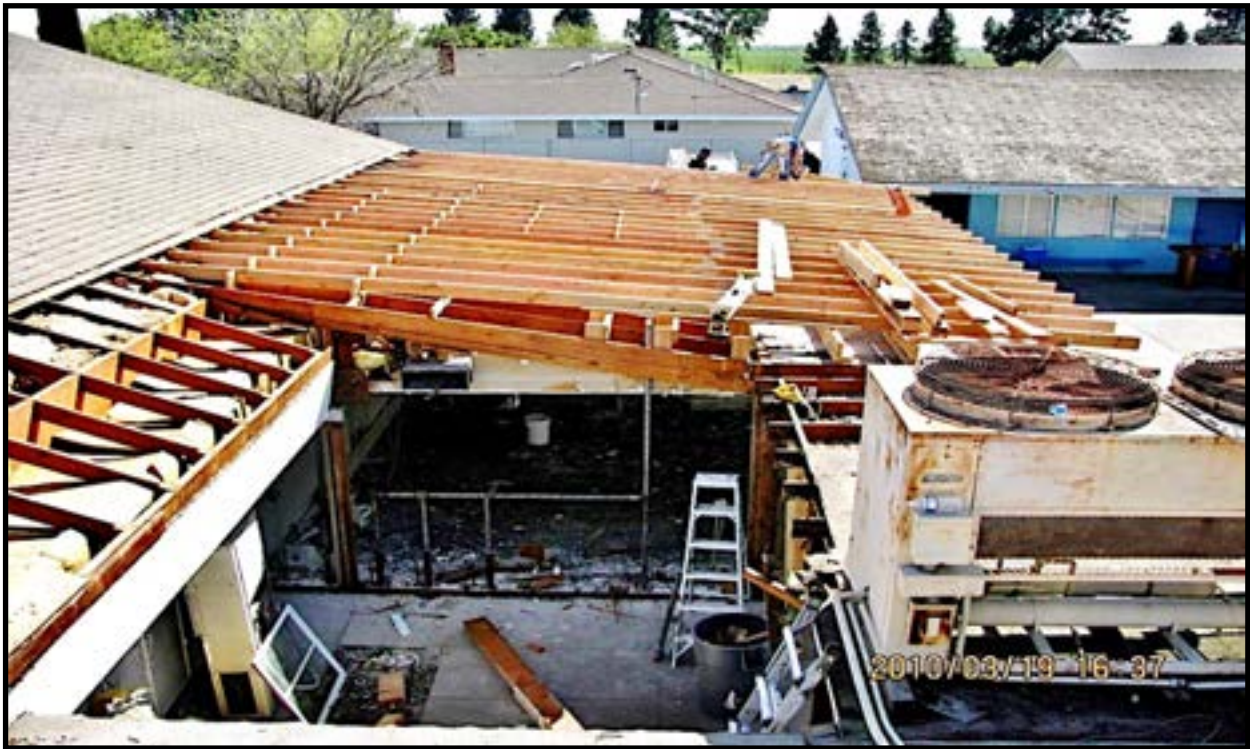
Renovation work continues on Saint Anne Church
