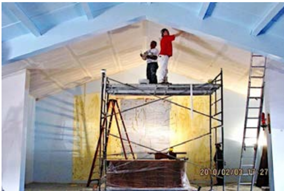
Renovation work begins on Saint Anne Church
