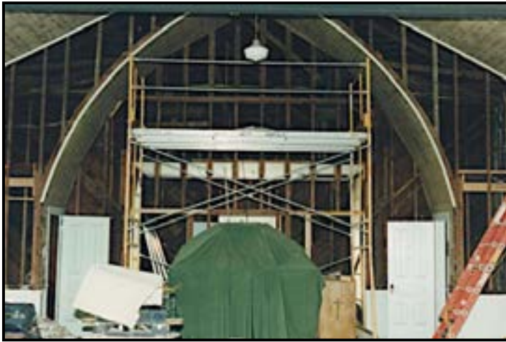
Interior Renovation, Saint Agnes Church, May 8, 2003
